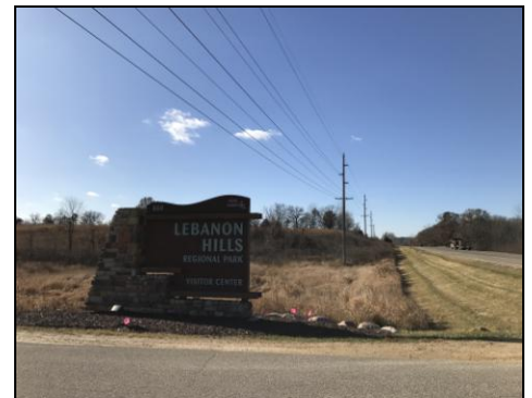
Transmission lines to be rebuilt and requested location of new easement along Cliff Rd.
